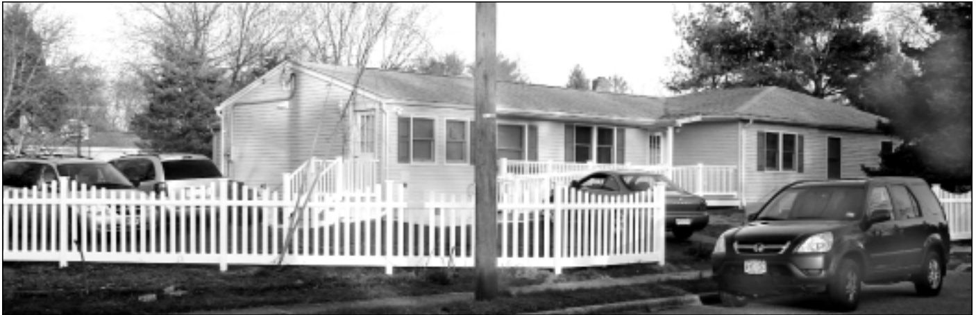
Renovations to AMIB's sixth group home — our first home outside Ocean County — were recently completed, and the first resident has moved in. AMIB is grateful to the donors listed here whose generosity has helped us complete these renovations.
